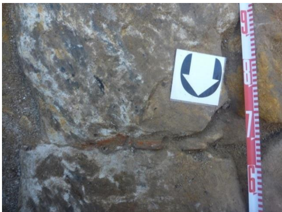
Figure 2.17 A detail in footing [200] showing the use of terracotta tile fragments for packing between the stone block joints. (Source: GML 2013)
