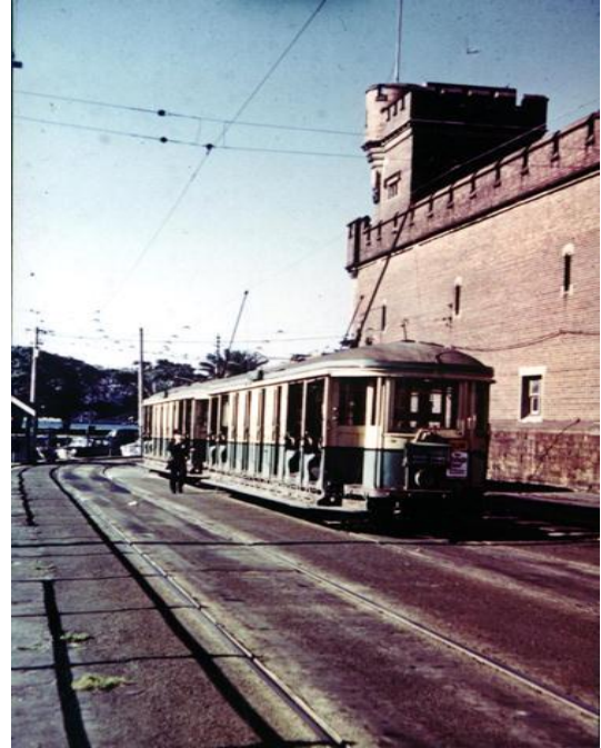
Figure 2.6 Western external side of the Tramcar House with sandstone foundations to ~1.5m. (Source: City of Sydney Archives 044/044475)
