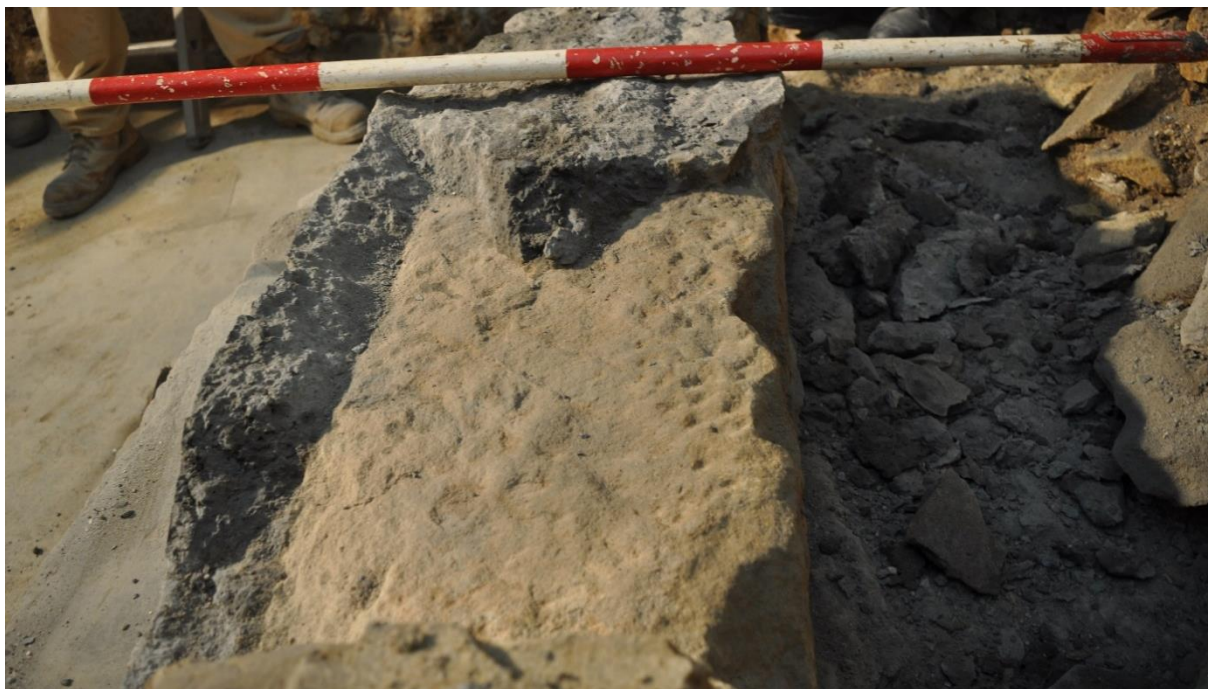
Figure 3.13 Excavation phase 2—The concrete steps [15] were cut (removed) from the sandstone steps [16], revealing the picked sandstone blockwork [21] of the earlier steps. (Source: GML 2019)
