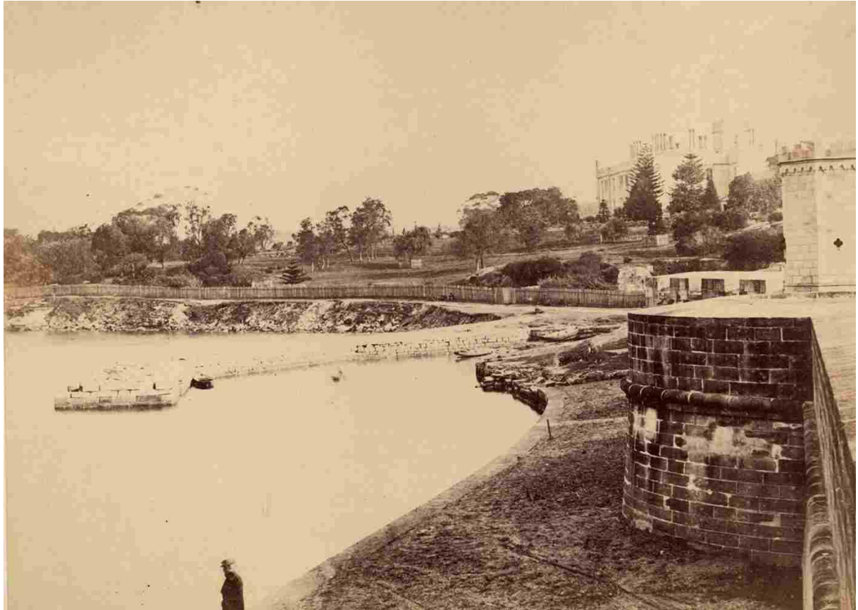
Figure 2.4 Eastern side of Fort Macquarie, facing south, showing the height of the external buttress ashlar sandstone wall, and the low seawall, with the esplanade defining the extent of land reclamation. (Source: State Library of NSW, FL1227860)
