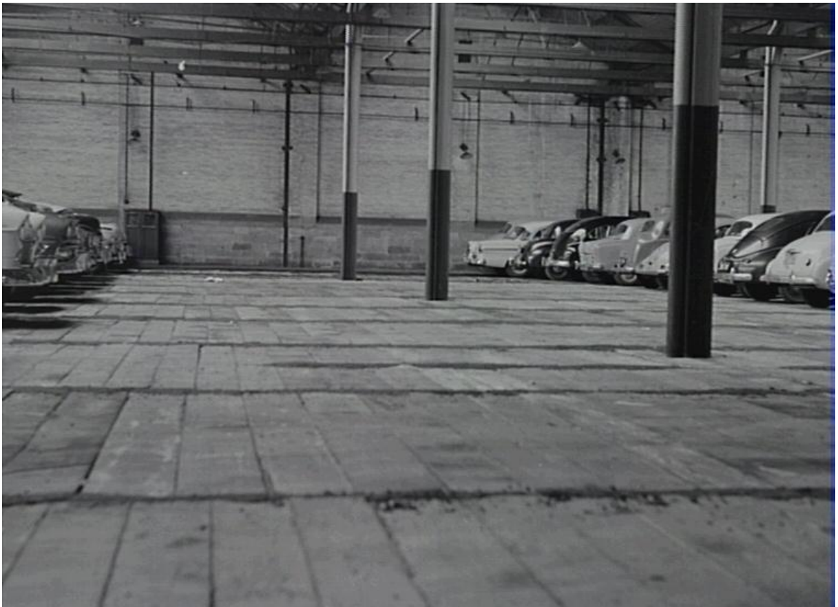
Figure 2.7 Internal view within the Tramcar House following closure of the tram system and use as a carpark. The floor is either wooden or concrete slats. The external lower sandstone wall is clearly visible at the height of the car roofs. (Source: City of Sydney Archives 101/010405 NSCA CRS 48-405)
