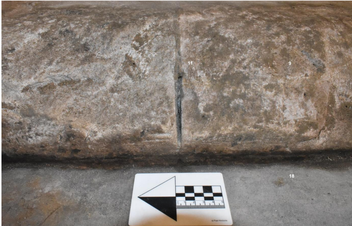
Figure 3.11 Excavation phase 1—Modifications to the sandstone wall [9], with cut-and-fill with concrete [11]. The rough chamfering to create a curved edge is evident. A wear line in the sandstone parallel to the concrete surface can be seen. (Source: GML 2018)
