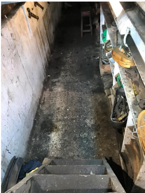
Figure 3.16 View down the stairs into a tram service pit. The wall height is around 1m. (Source: GML 2018)
