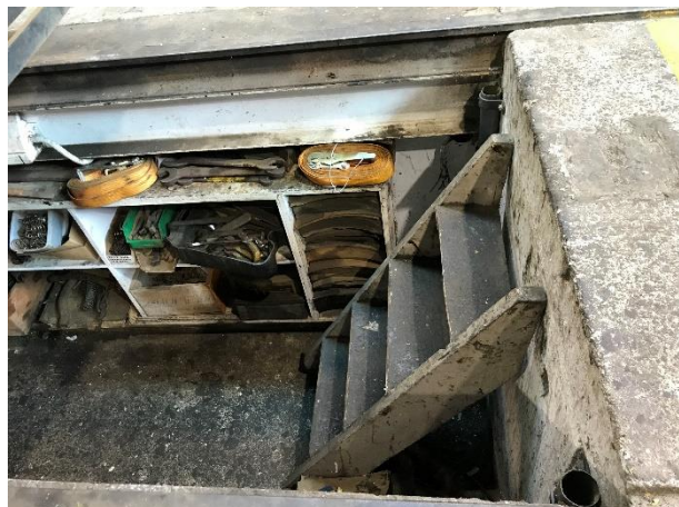
Figure 3.17 Tool storage alcoves set into the wall of the service pit. (Source: GML 2019)
