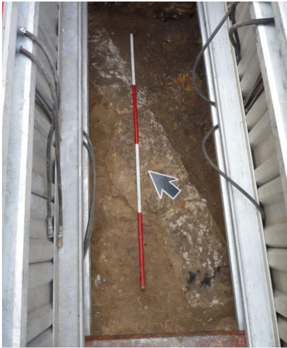
Figure 2.15 A section of sandstone footing [077] believed to be part of the Fort Macquarie buttress wall was revealed in the north section of the piling trench. Photo scale: 2m. (Source: GML 2012)
