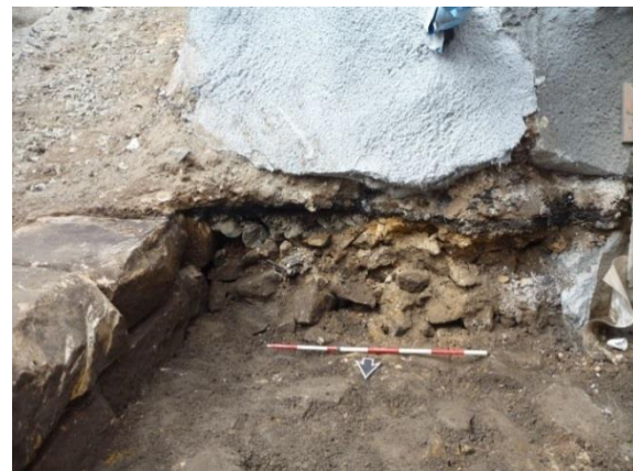
Figure 2.18 The south section of the substation exhaust plenum shows the reclamation rubble fill and the line of asphalt surface. Photo scale: 1.4m. (Source: GML 2014)
