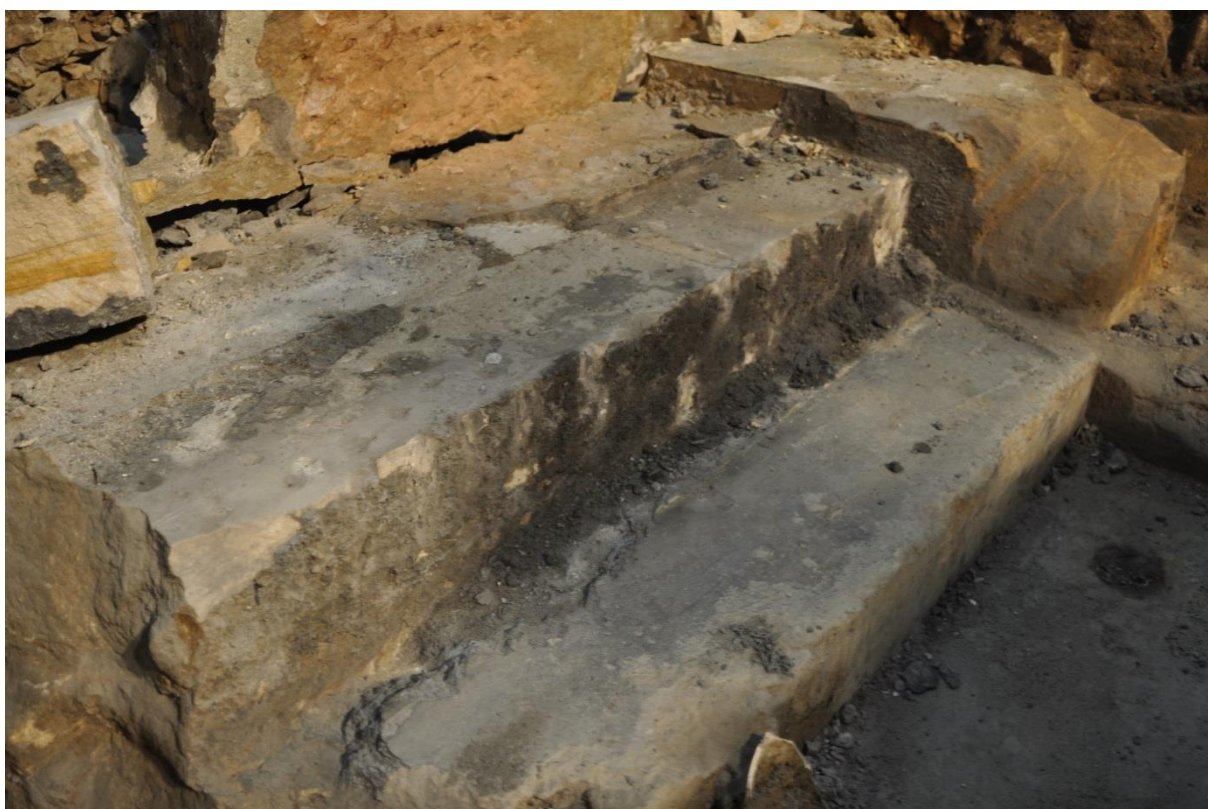
Figure 3.14 Excavation phase 2—The sandstone steps [16] were disassembled and comprised a number of distinct rectangular blocks, with some lime mortar binding. (Source: GML 2019)
