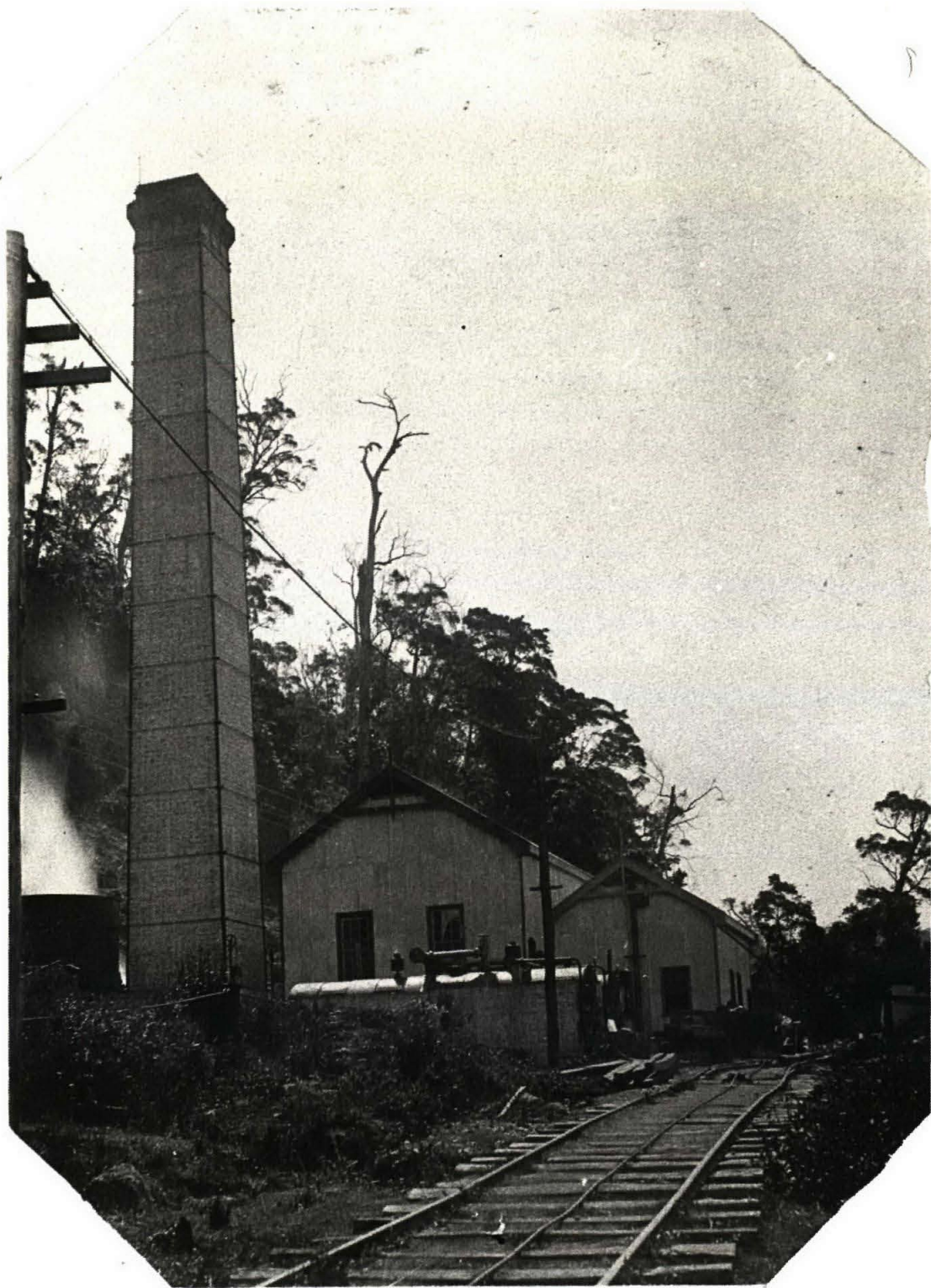
Terminus of new Railway to Fan Shi. Chimney, boilers for Engine House, and Electrical Engine Power House. Power cable can be seen overhead - to left of view.
