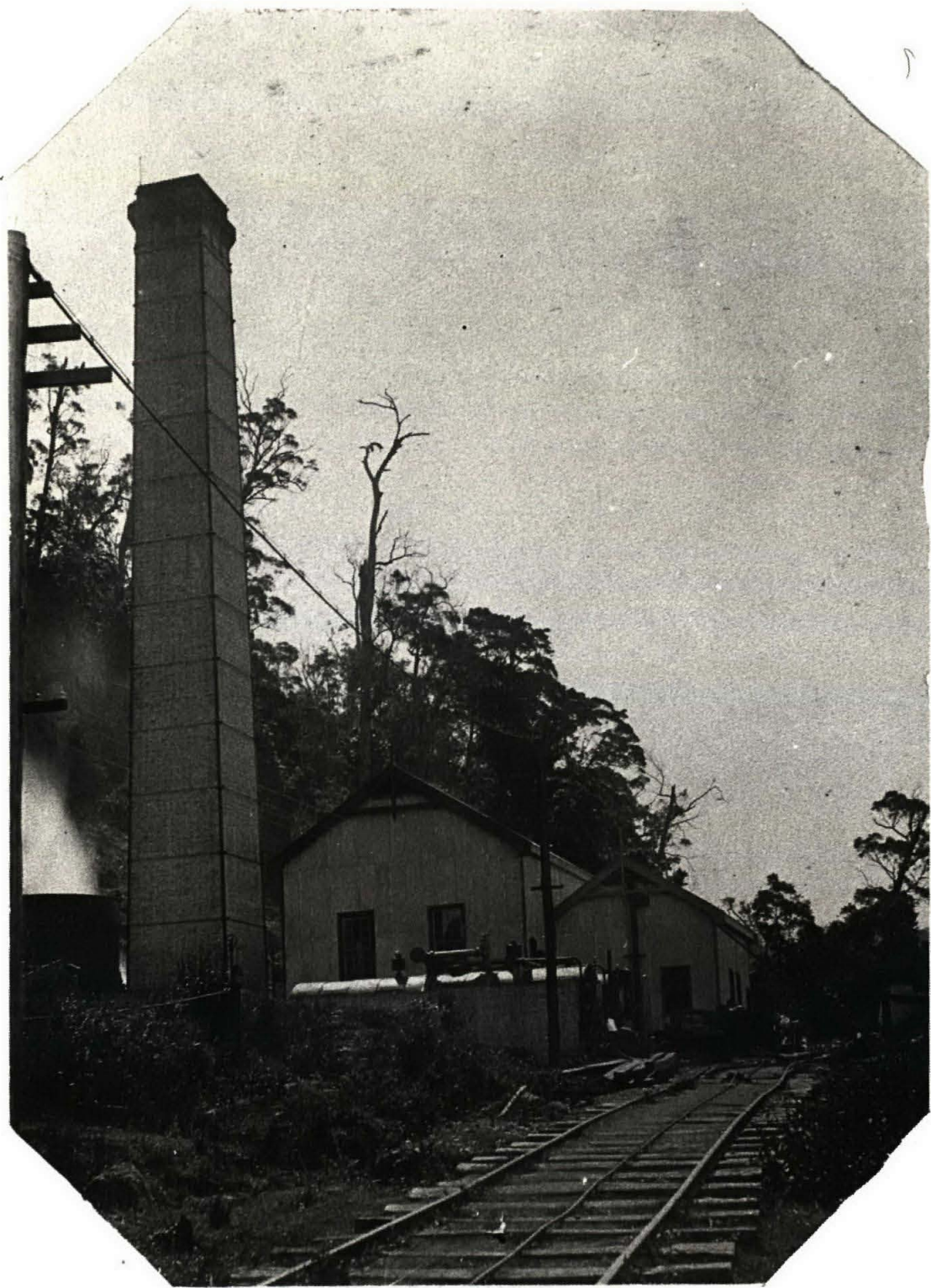
Terminus of new Railway to Fan Sit. Chimney, boilers for Engine House, and Electrical Engine Power House Power cable can be seen overhead - to left of view.
