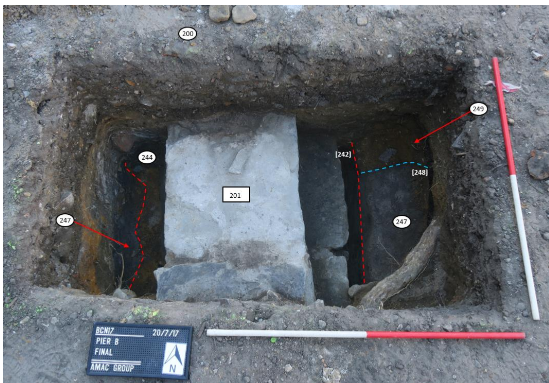
Figure 3.25 Pier B – showing sandstone footings [201], facing north. AMAC Group (20/07/2017, IMG_1141)
