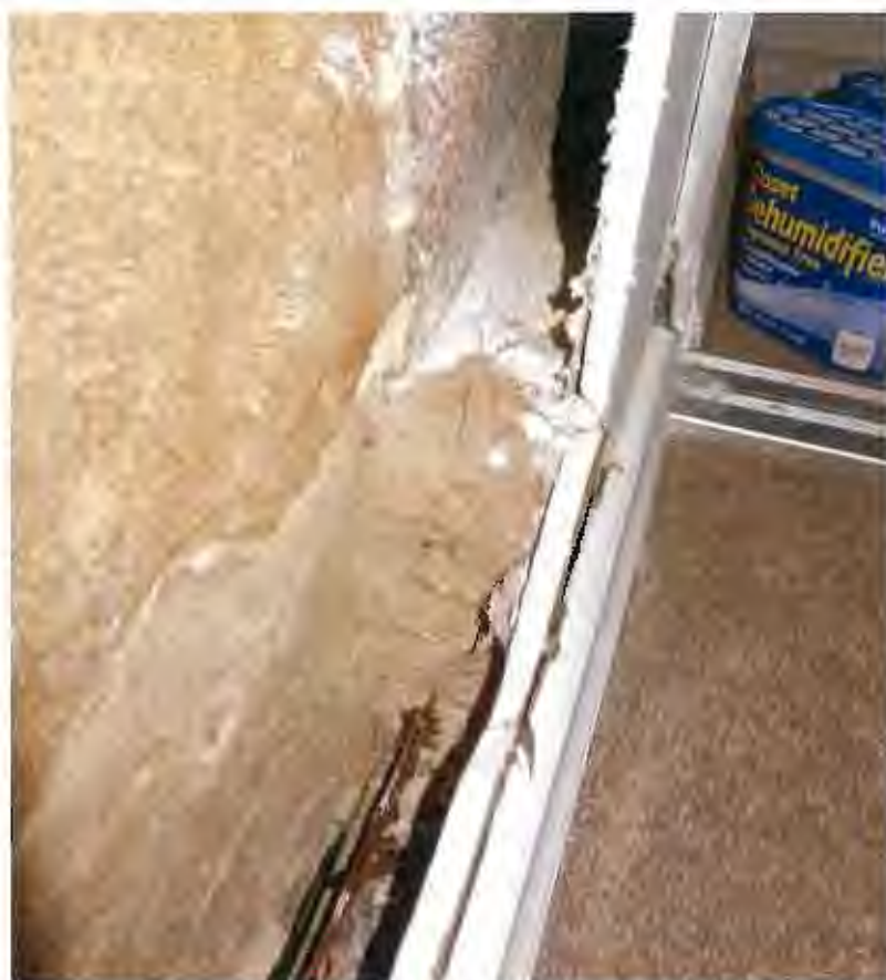
Figure 11 Opening 5 in Unit 3, which is against an external wall. Note the damp sand that has accumulated behind the plasterboard. Vacuuming out the debris in the foreground has revealed the substantial depth of sand, and the rusting steel channel at the bottom, which sits on the concrete slab floor. To the left of the rusting channel is the black plastic membrane that is intended to protect the concrete from dampness. This area was not treated in 2013.
