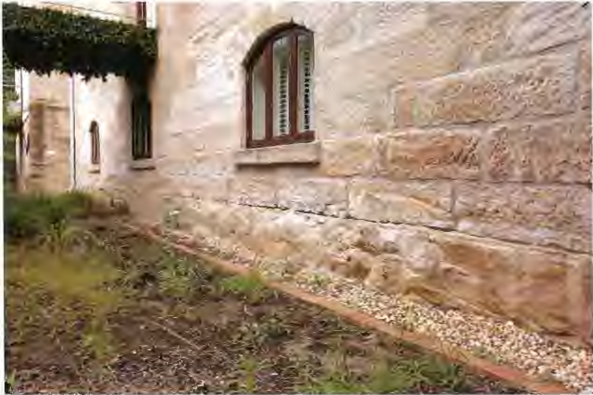
Figure 4 North wall showing the bottom 'course' of sandstone, which is actually natural bedrock. An attempt to divide it into 'stones' has been made by cutting narrow slots and filling them with mortar.
