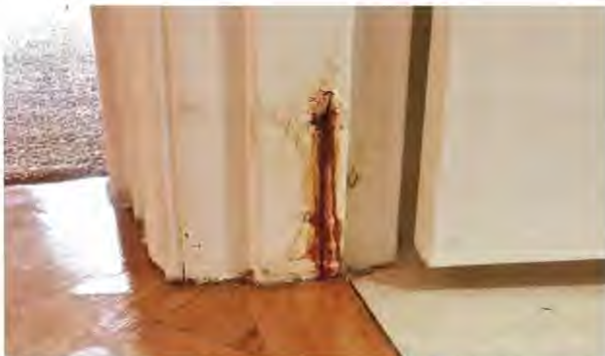
Figure 6 Corrosion (rusting) of steel bathroom door frame due to moisture from behind, Unit 3. Similar corrosion is apparent in Unit 1.
