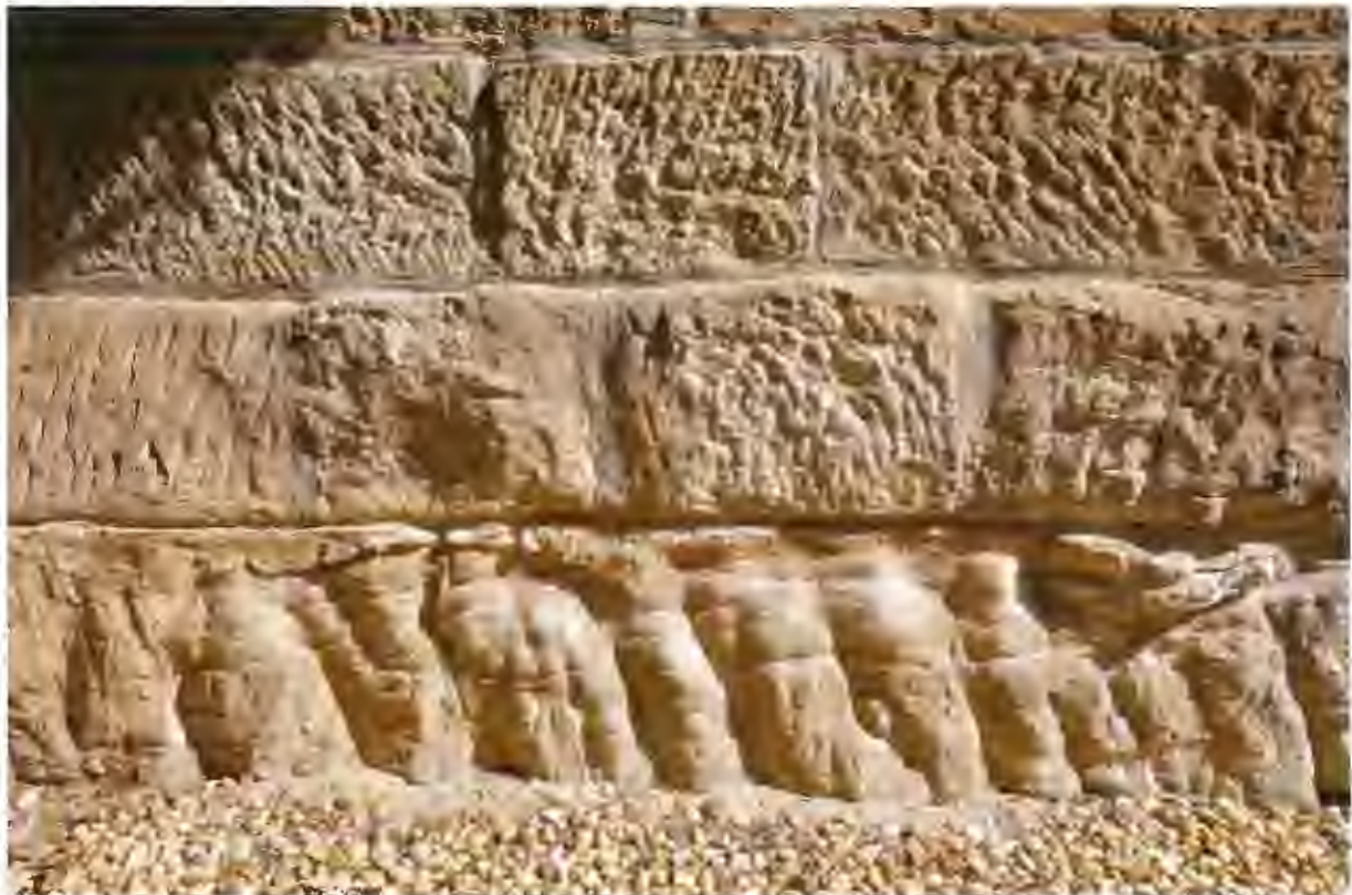
Figure 2 Fretting of the sandstone bedrock of the north wall due to salt attack and rising damp, with sand accumulating in the pebble bed below. Note the mortar patching of some stones at the left.
