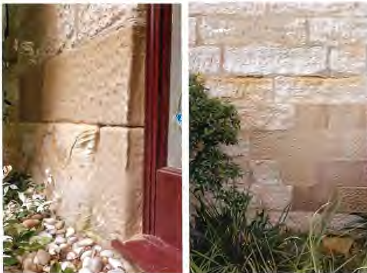
Figures 3 and 4. New stone inserted in 2002 has a pale brown colour compared to the original whiter stone. At left, the new stone is decaying, as is the mortar-patched bedrock below and to its left. On the right, decay of two original stones is made worse by the impermeable nature of the cement-lime repointing, the stones are retreating from the mortar which now stands proud, leaving a shadow line.
