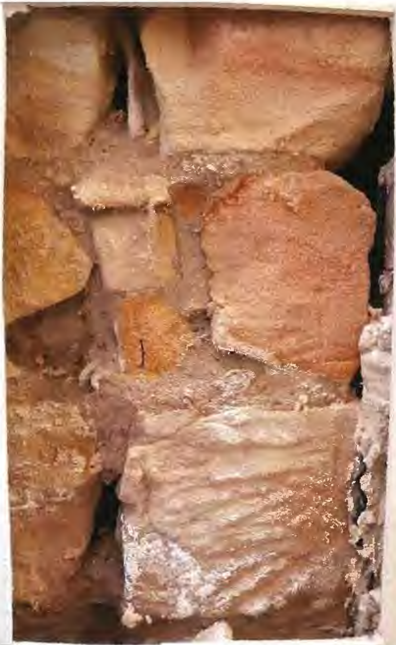
Figure 8 Opening 2 in Unit 1, showing a cross section of about two thirds of the width of an internal sandstone wall. Note salts on surfaces of all stones, particularly the lower ones, and the decay of the mortar from between the stones.
