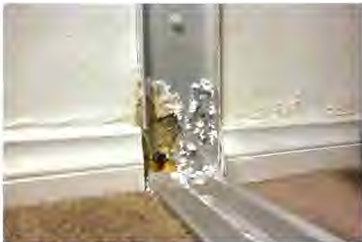
Figure 5 Corrosion of aluminium sliding wardrobe door frame due to salts and to dissimilar metals (Unit 3). Early stages of corrosion of the same aluminium detail can be seen in Units 1 and 2. Also note typical bubbling and blistering of paintwork due to moisture and salts. See also Figure 11.
