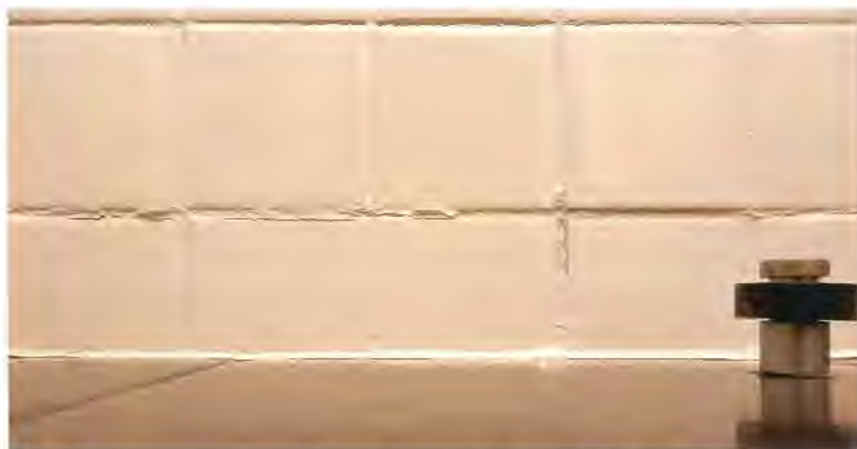
Figure 7 Decay of grout between bathroom tiles in Unit 1, due to salt attack.
