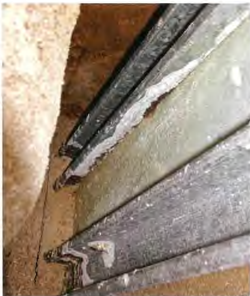
Figure 10 Opening 6 in Unit 3, looking down the gap between salty stone at left and the galvanised steel frame that supports the plasterboard lining at right. Note how the almost hidden U-section channel at the base is full of sand. Corrosion of the zinc galvanising (white) has lead to brown rusting of the steel beneath. The inner surface of the grey-green plasterboard is speckled with white salts.
