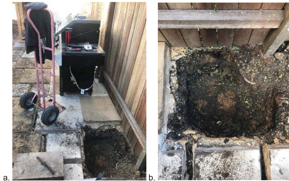
Figure 3.28 Hole 3 – excavation of topsoil – bedrock exposed a. Facing south b. facing southwest. J.Baloh, 14/07/17
