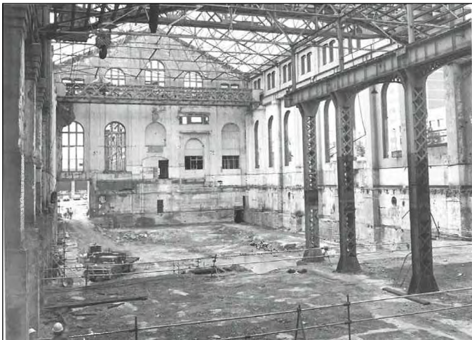
c.1968 Image of the main powerhouse volume, noting the severe dilapidation and the state of the powerhouse as a disused space, demonstrating that the original working fabric was already not intact and only in a reasonable condition.
