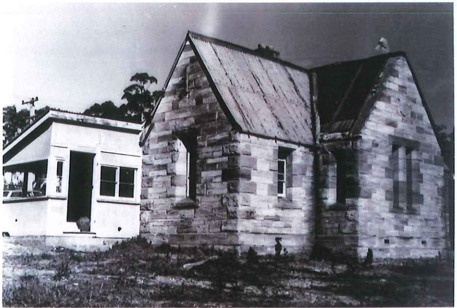
Photo 21: View from the north east, showing the rear fibro additions of the 1950's – since demolished.
